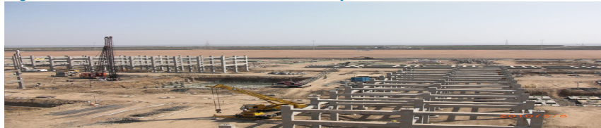
Figure 3.3: OPaL construction site at Dahej
